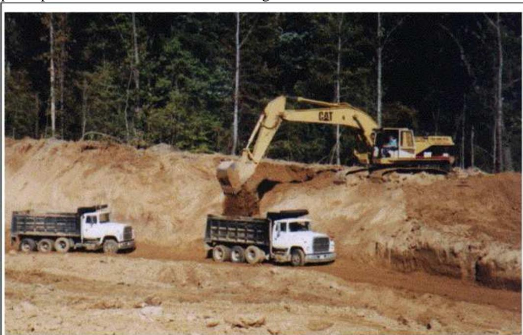
Figure 1: Excavator loading a truck in a mass excavation scenario. The excavator sits on top of an elevated bench, removes the material from the bench, and deposits it into the back of the truck.
