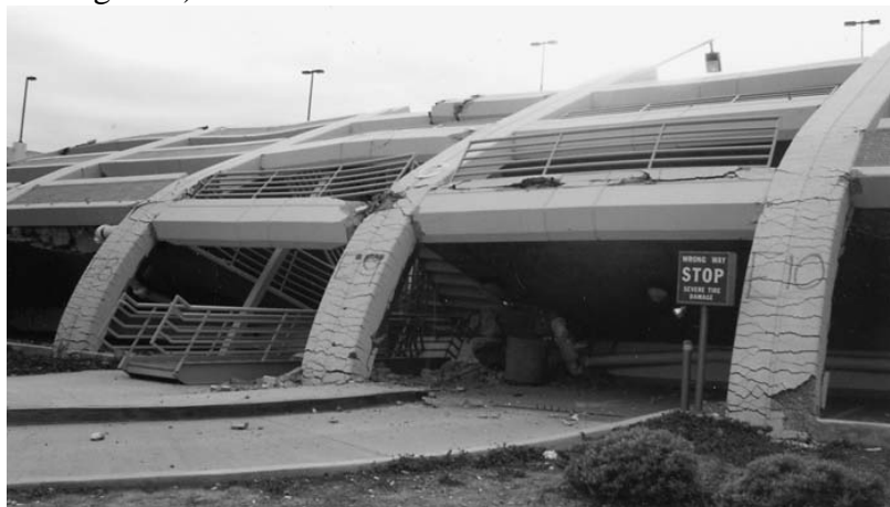
Figure 1. Parking structure that collapsed during the 1994 Northridge earthquake, California State University, Northridge Campus.
